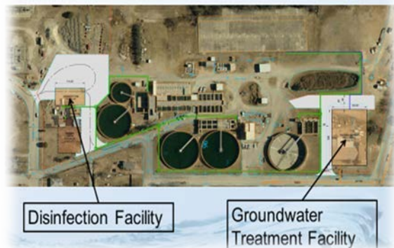
Ground Water Treatment Facility
