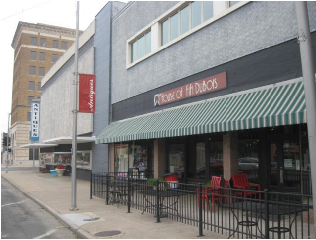
South of building (House of FiFi Dubois)
