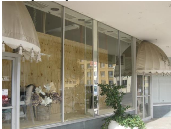
Existing awnings and entrance
