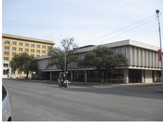
North of the building
