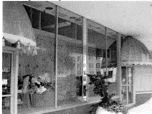
Existing awnings and entrance
