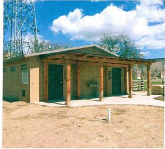
Pre-cast concrete restroom
