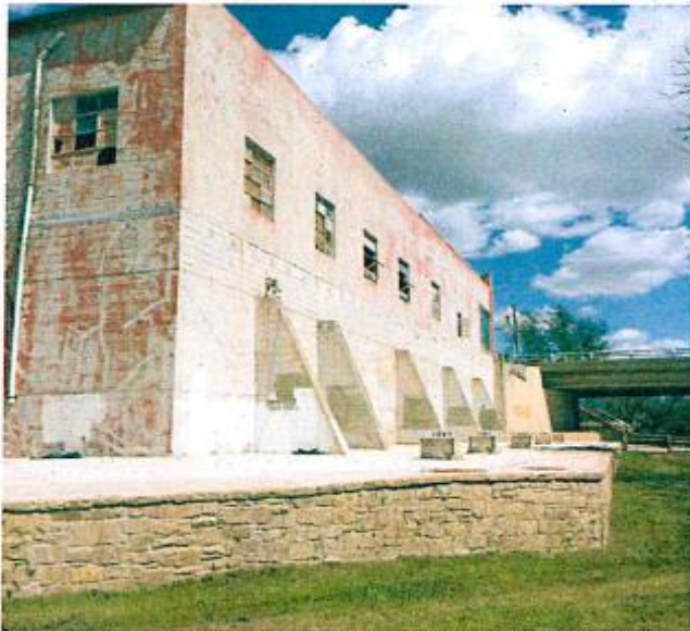
Adjacent Building to the north
