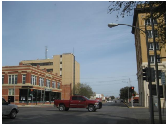
Northwest of Building
