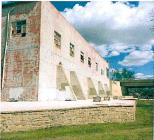
Adjacent Building to the north
