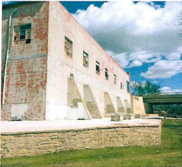
Adjacent Building to the north
