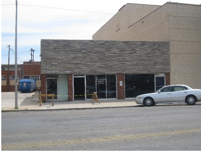
North Elevation – Turner Building 109 West Beauregard Avenue
