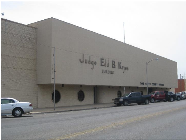
North Elevation – Keyes Building 113 West Beauregard Avenue
