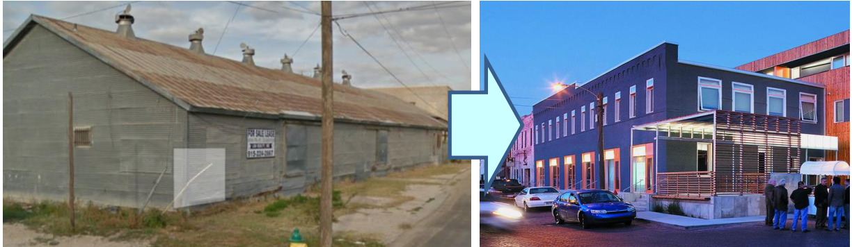
Example 1: W. 4th Street Warehouse Site
