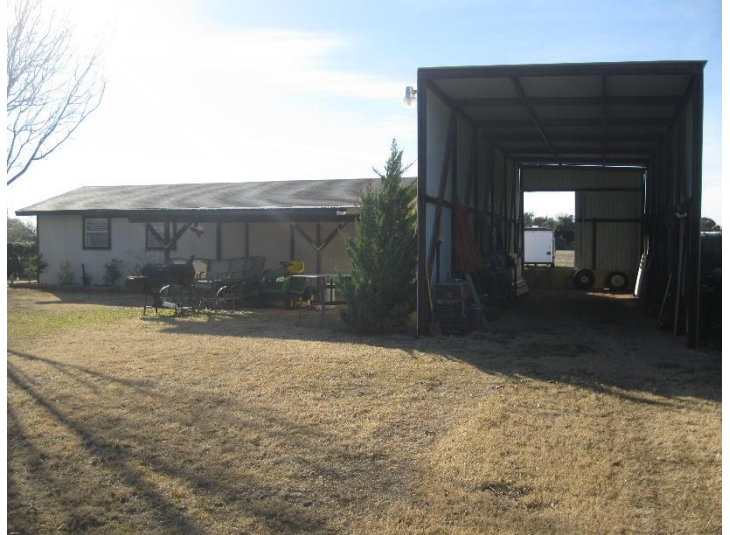
Existing Workshop Building and RV-port
