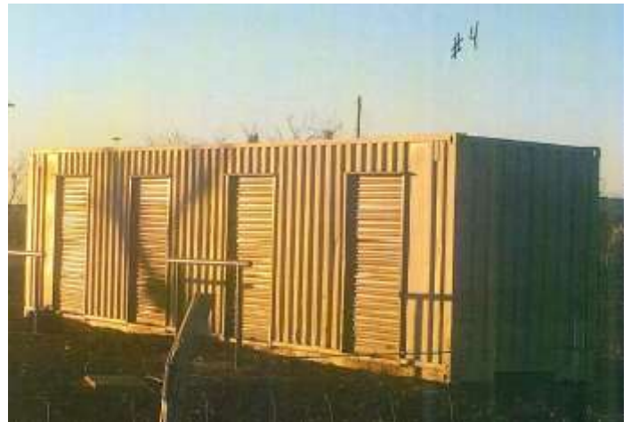
Existing shipping container (to be removed)
