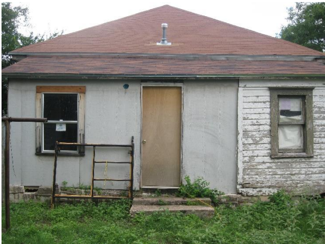
Rear of Existing Home
