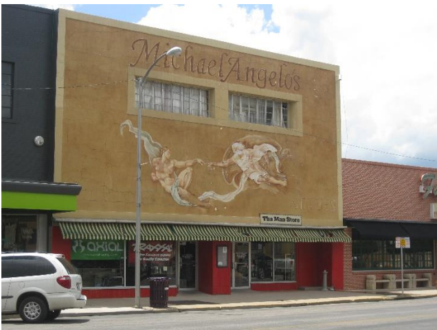
Facades North of Building
