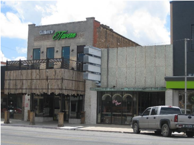
Facades South of Building
