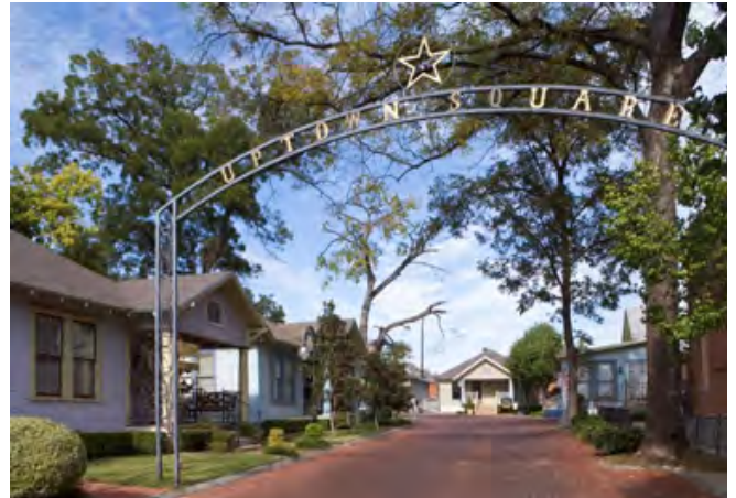
Cottages picked up and relocated into clusters around bricked parking court
