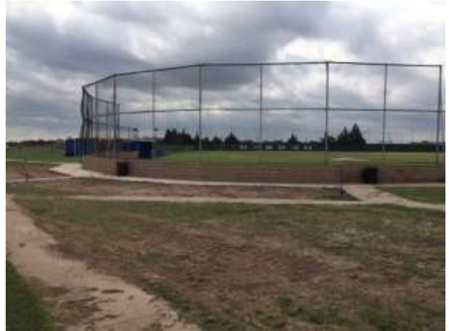
Looking east elevation
