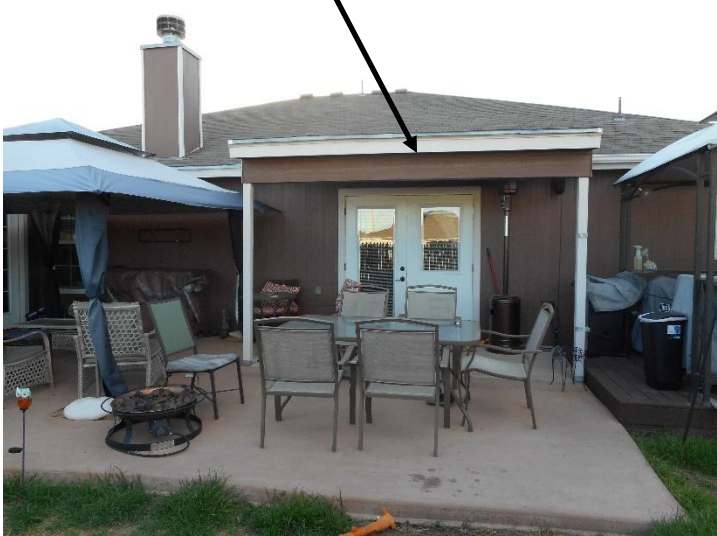
Existing porch (to be removed)
