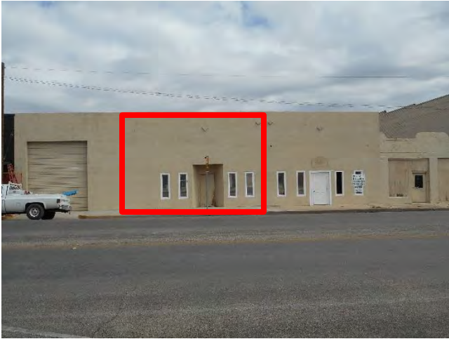
Existing façade looking east
