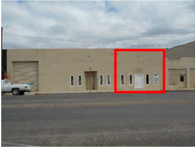
Existing façade looking east
