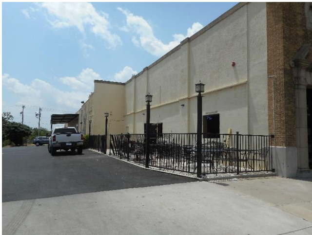
South at Subject Canopy Area
