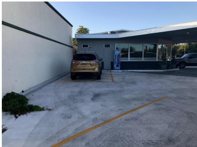
No-parking area behind sign (striped)
