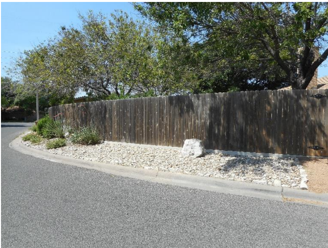
SOUTHEAST EXISTING PRIVACY FENCE
