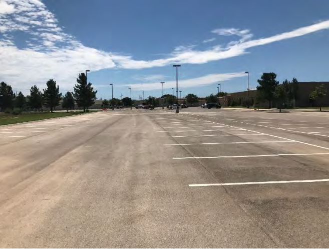
EXISTING REAR PARKING AREA
