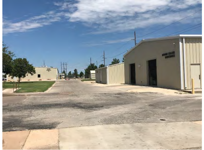
CLOSE UP – EXISTING METAL BUILDINGS
