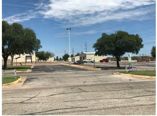
NORTH AT EXISTING METAL BUILDINGS
