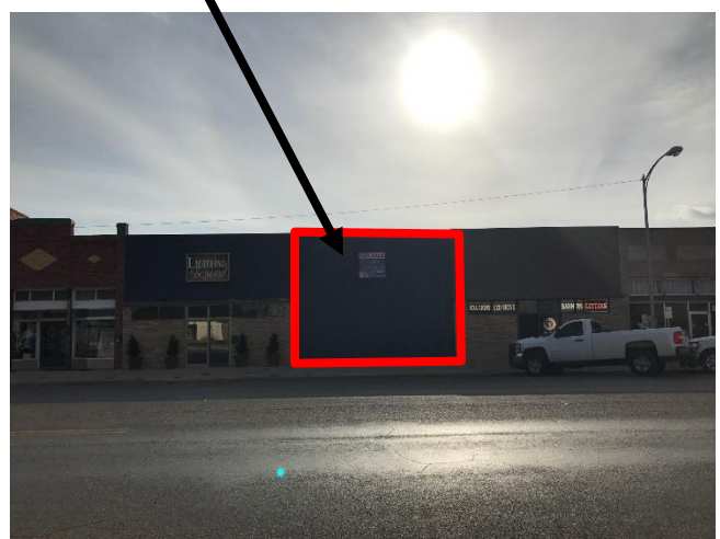
EAST AT PROPERTY
