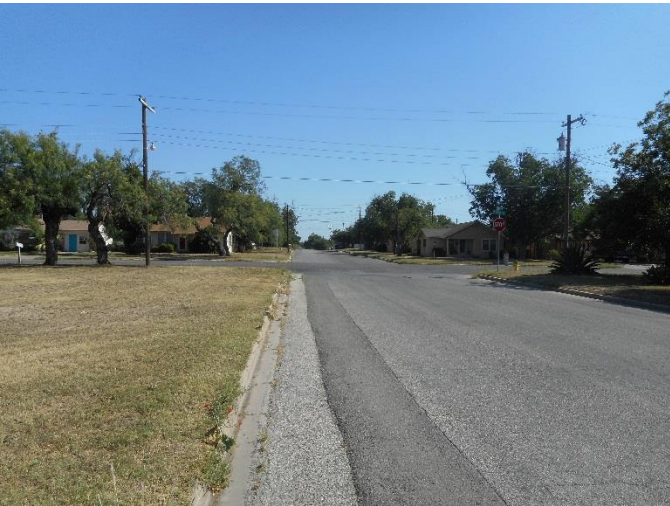
LOOKING NORTH ON ARCHER
