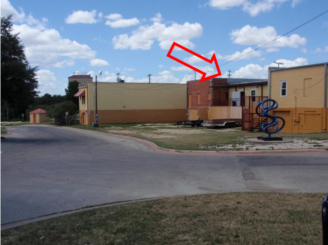
North toward Rear of Building
