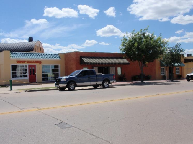
Front of Building
