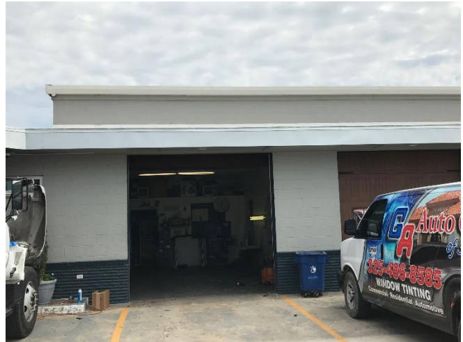
MAIN BUILDING GARAGE FACING WASHINGTON ST
