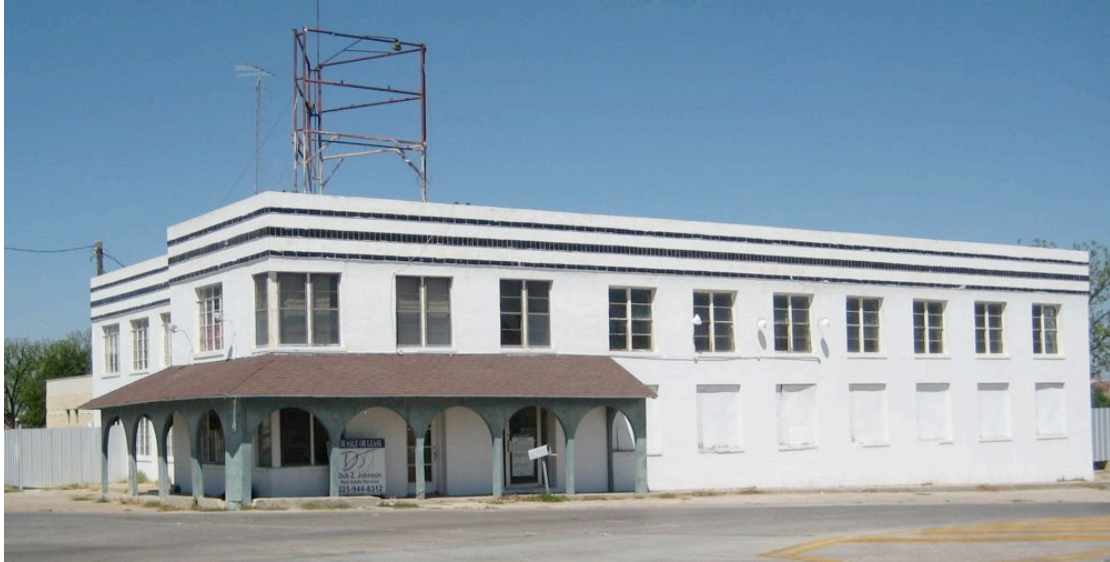
Figure 5-5. Banner Creamery Factory and Warehouse, built between 1931 and 1949.
