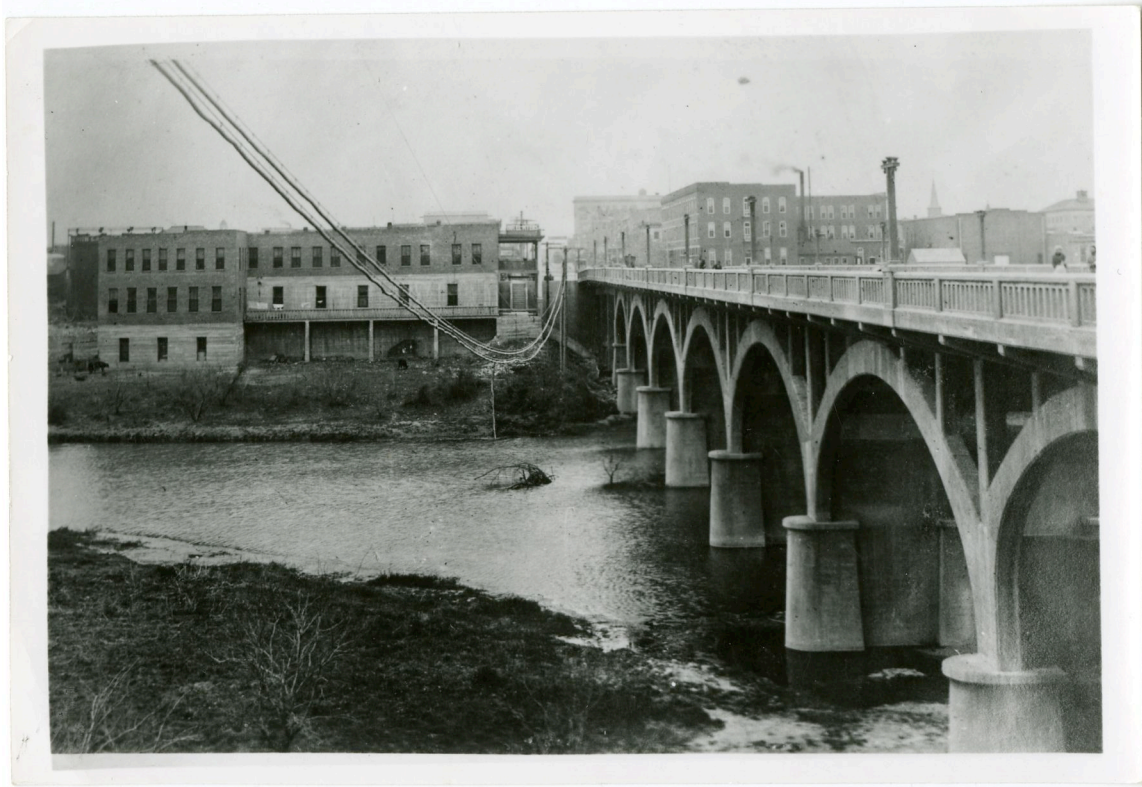
Figure 3-7. Chadbourne Street Viaduct, Completed in 1913. Courtesy of West Texas Archives, Angelo State University.
