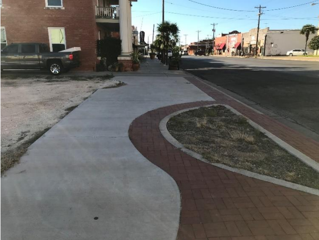
EXISTING SIDEWALK AND BRICK PAVER
