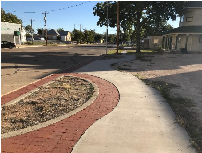
EXISTING SIDEWALK AND BRICK PAVER
