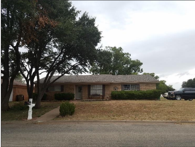
FRONT ON OLD POST ROAD
