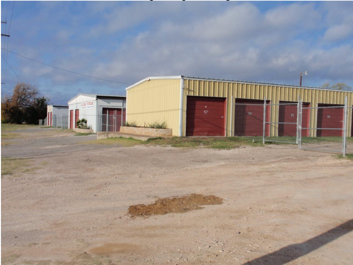
Existing Storage Buildings
