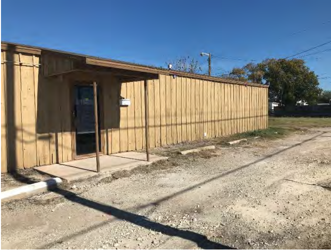
NORTH AT BUILDING
