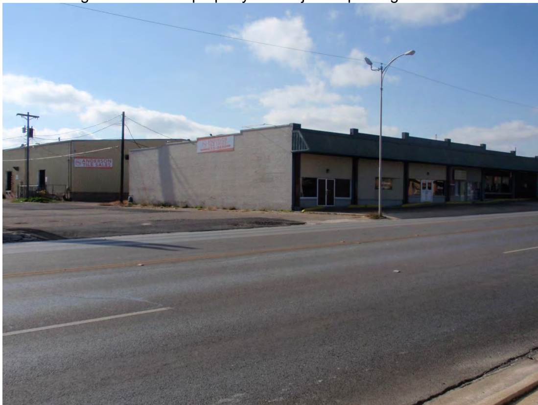
Lookgin south at the property and adjacent parking lot to the east
