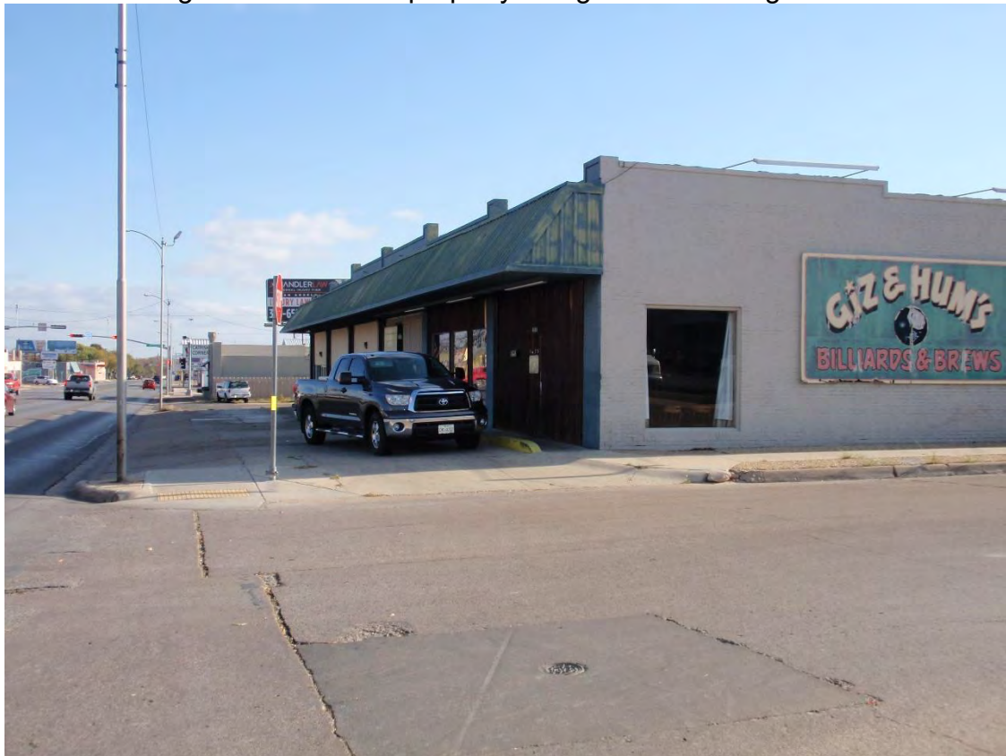
Looking northeast at the property along West Beauregard Avenue
