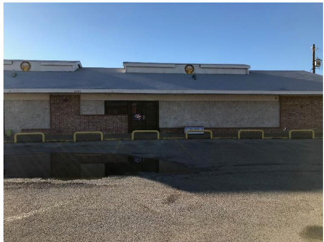
WEST AT PROPERTY (MAIN BUILDING)
