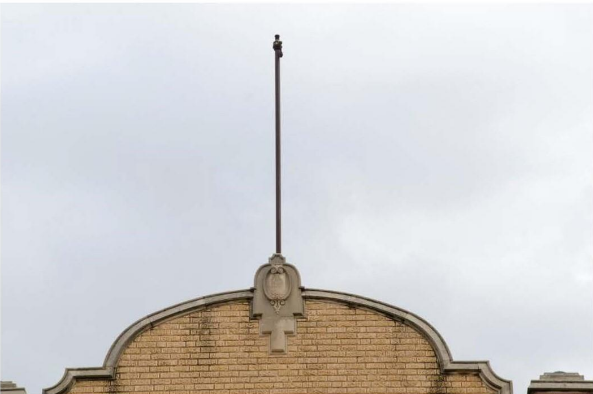
Photo 16: Parapet detail, west elevation, looking east
