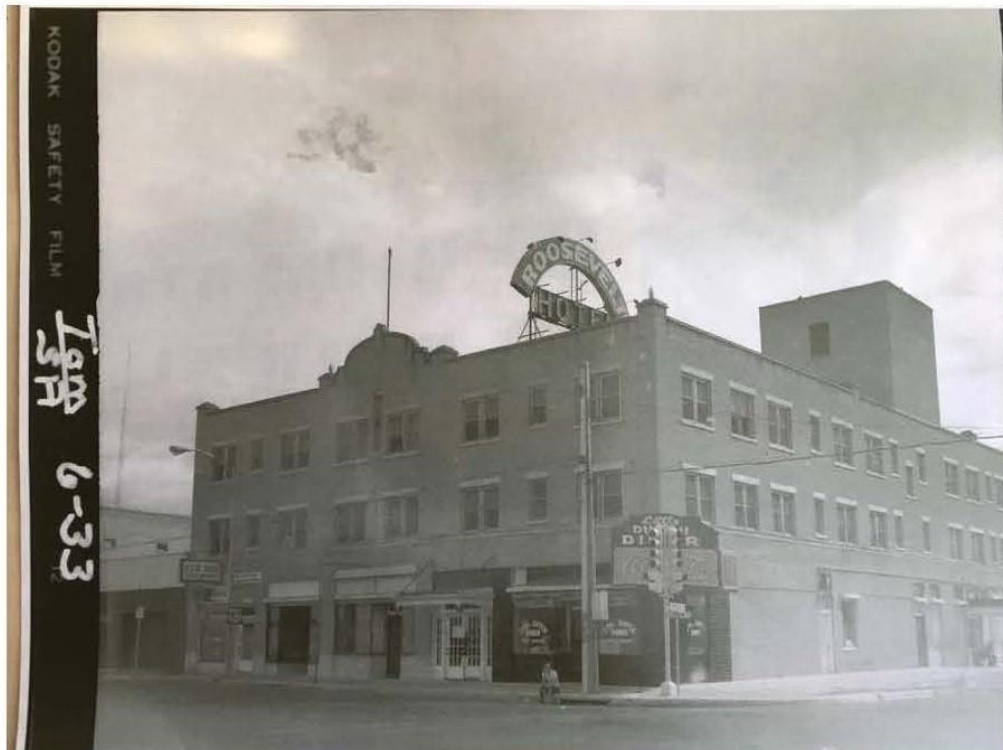
Figure 8: Roosevelt Hotel, looking northeast, Historic Photo – Undated
