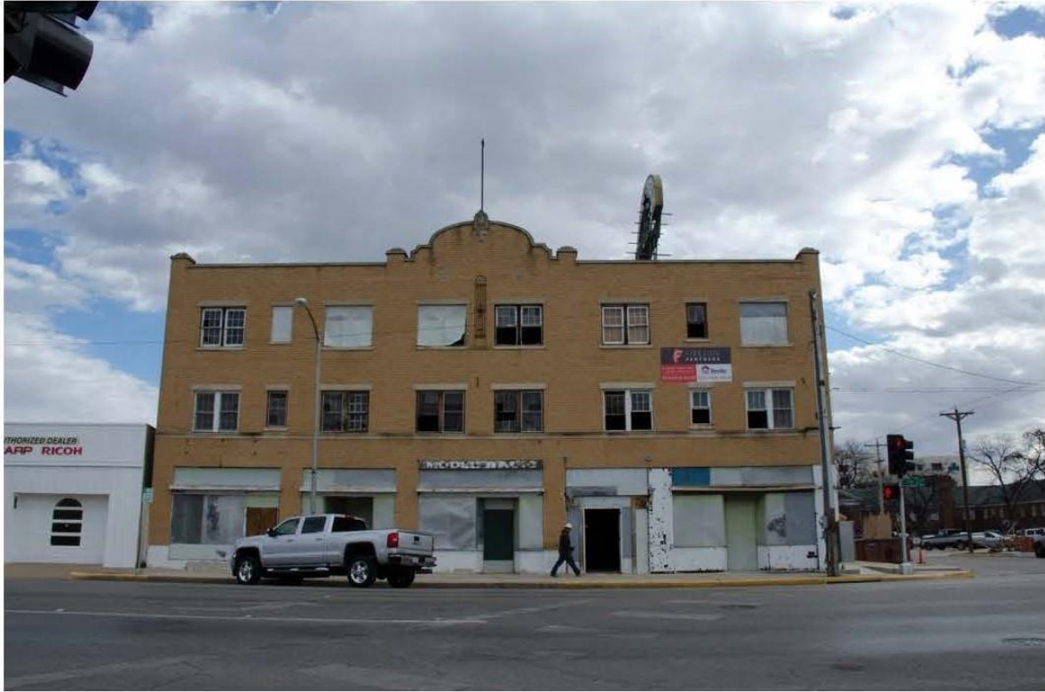
Photo 1: West elevation, looking east
