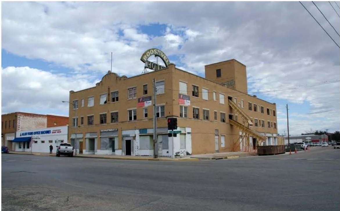
Photo 2: West and south elevations, looking northeast
