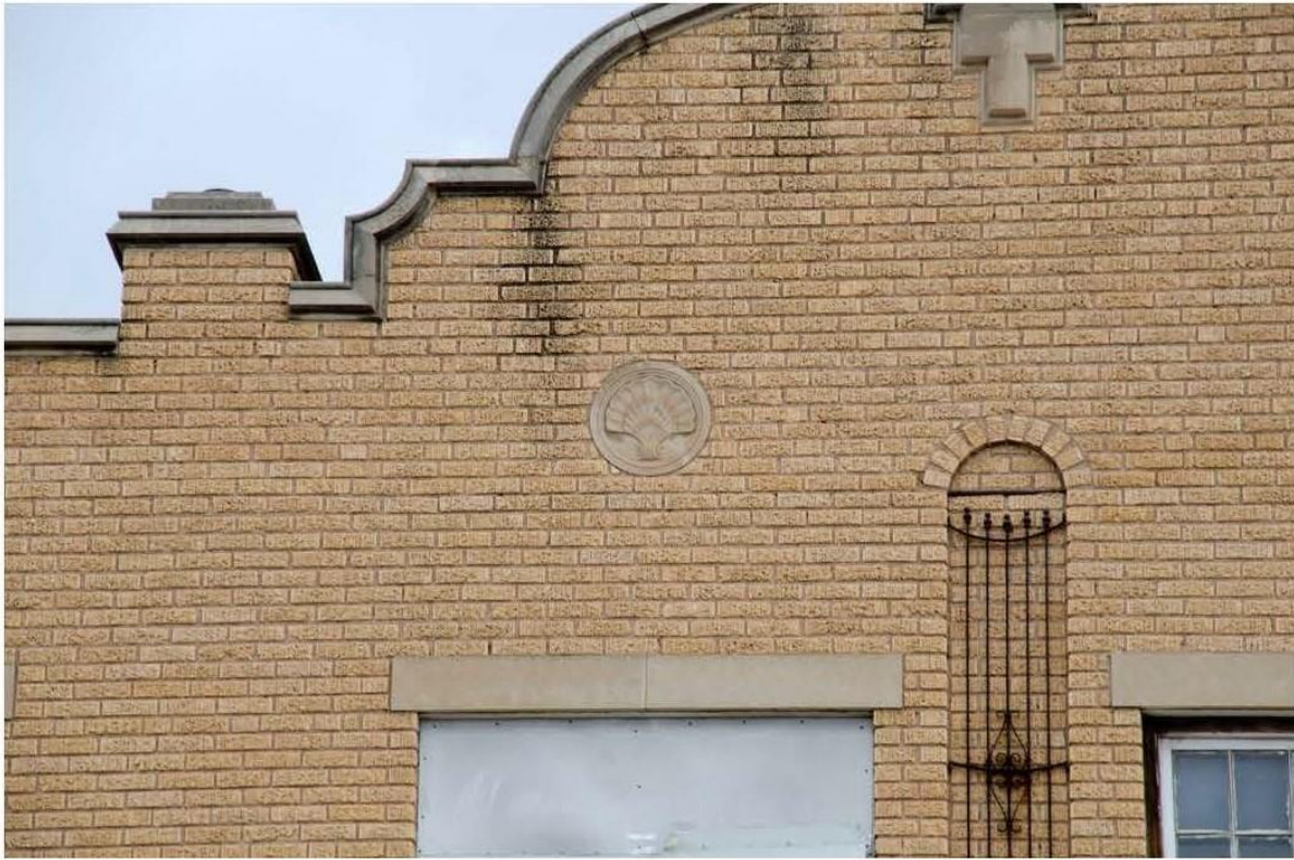
Photo 15: Masonry detail, west elevation, looking east
