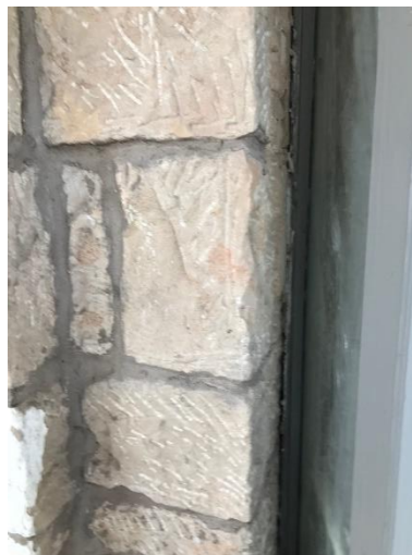
EXISTING FRONT FAÇADE ROCK (TO BE REMOVED)
