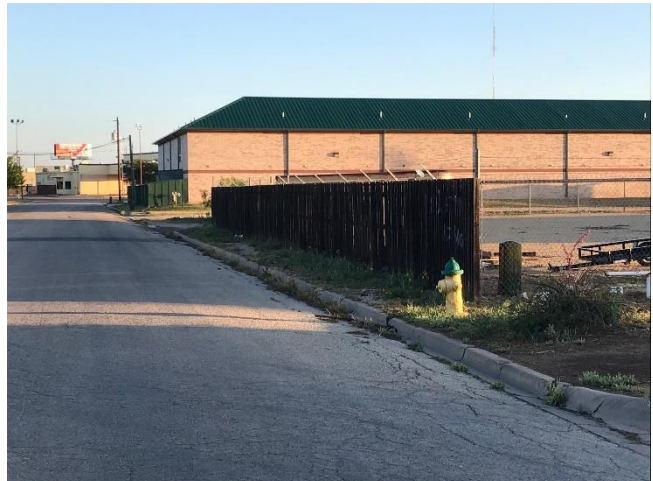
6-FOOT HIGH PRIVACY FENCE 2113 N. BRYANT BLVD. (ACTION PAWN)
