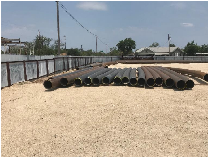
INSIDE PROPERTY LOOKING NORTH
