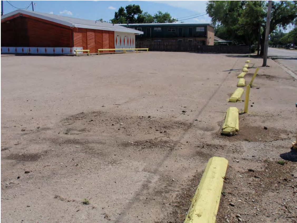
Existing Parking Lot Conditions North Side
