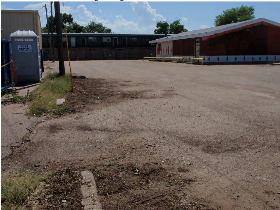
Existing Parking Lot Conditions South Side
