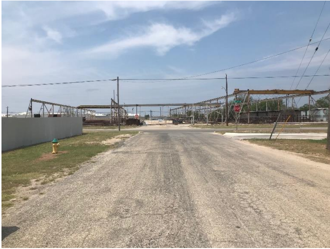
LOOKING WEST AT GRAPE CREEK ROAD
