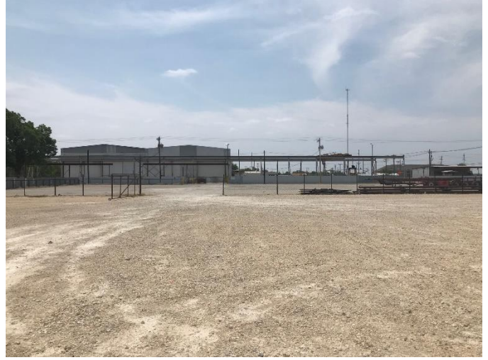
INSIDE PROPERTY LOOKING SOUTH
