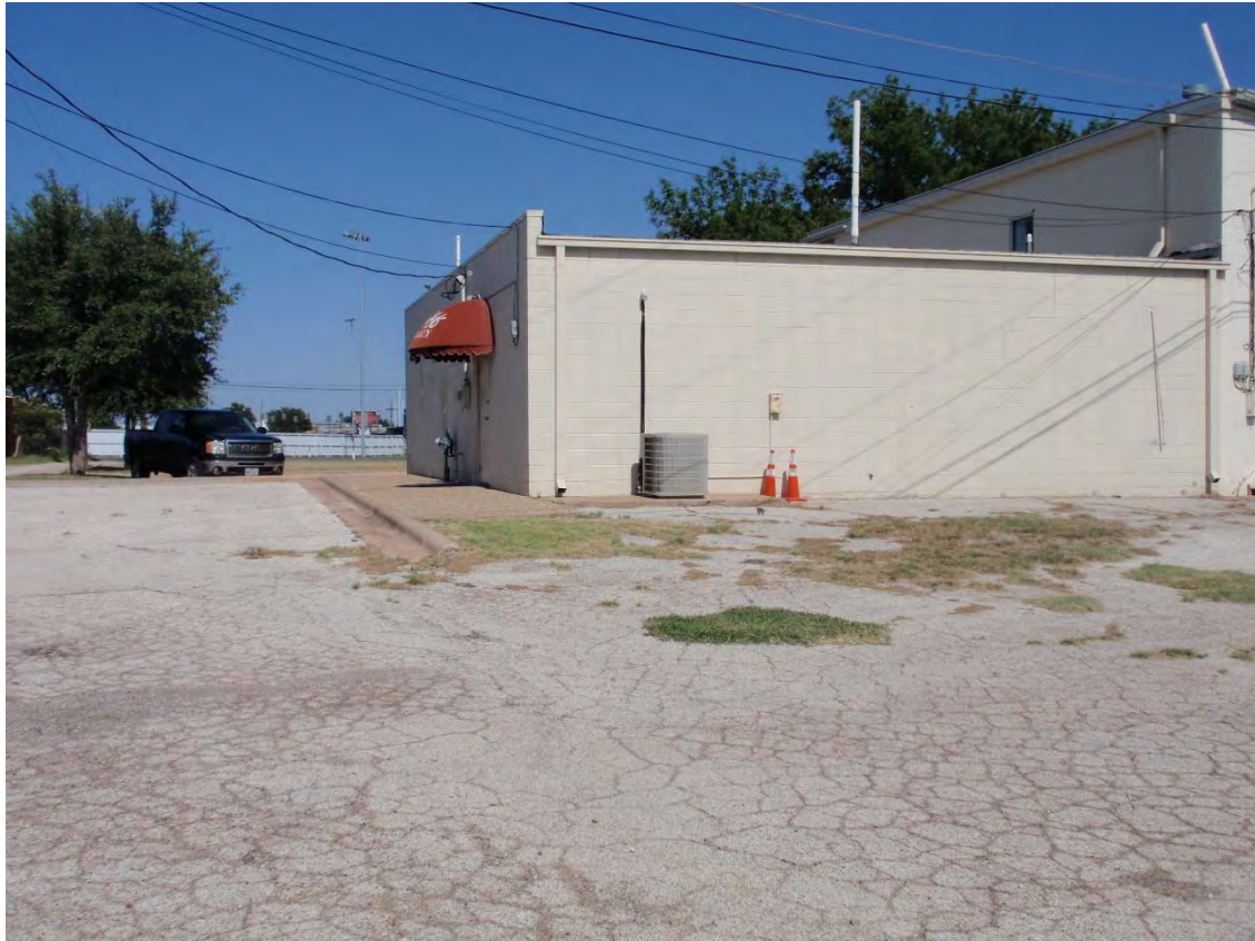
Back of Building Adjacent to Alley
