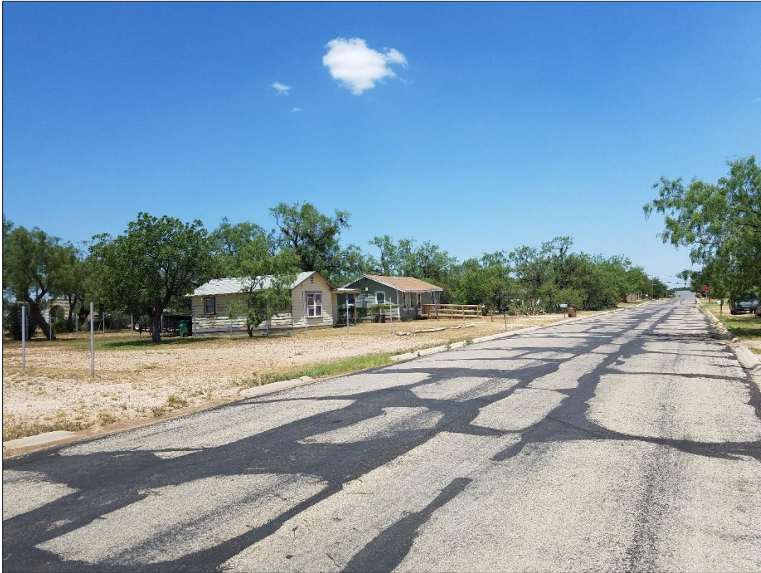
Looking East on Ben Ficklin toward Adjacent Vacant Lot and Residential Homes
