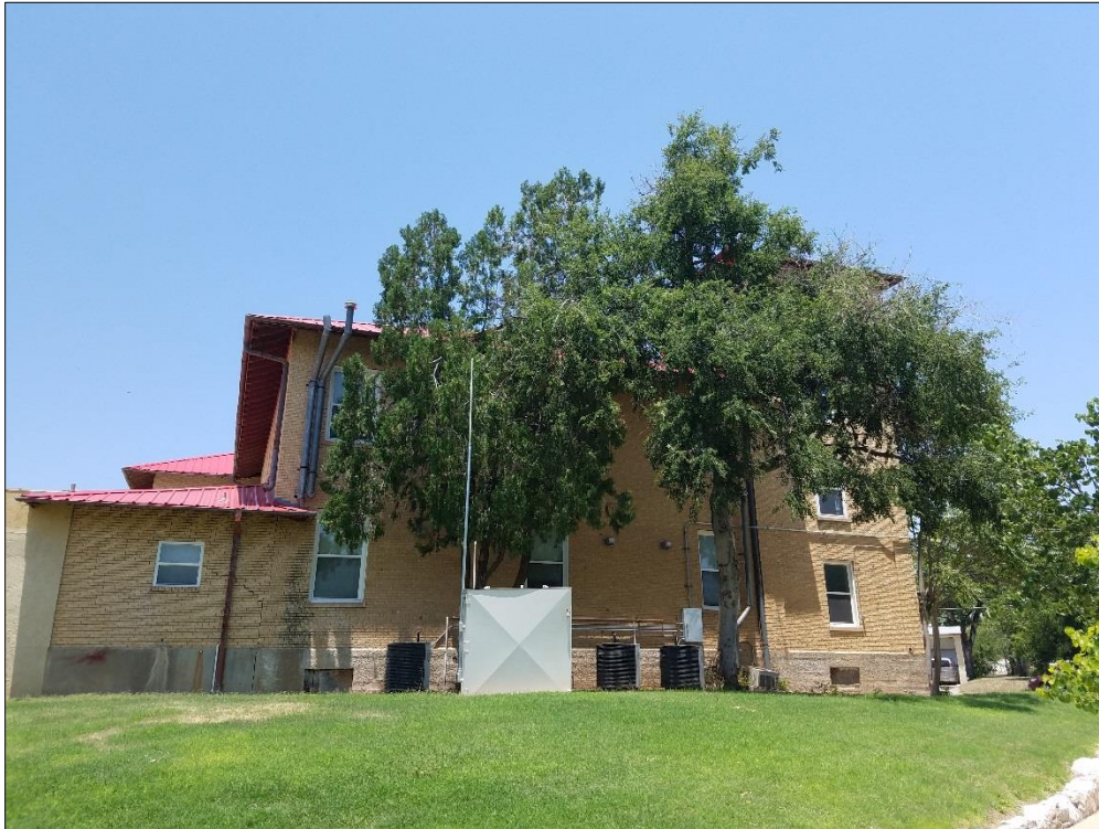
EAST ELEVATION (REAR OF PROPERTY)
