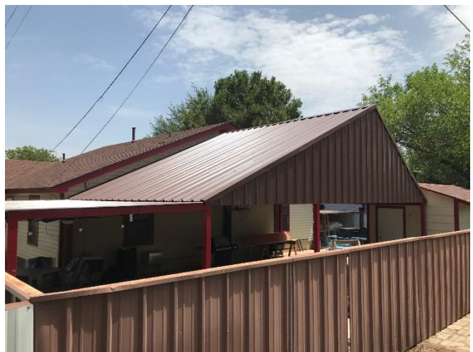
VIEW FROM REAR ALLEY
