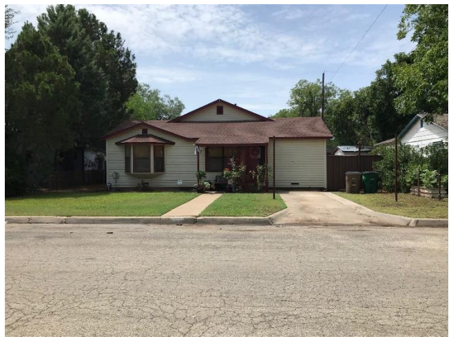
SOUTH AT SUBJECT PROPERTY (FRONT)
