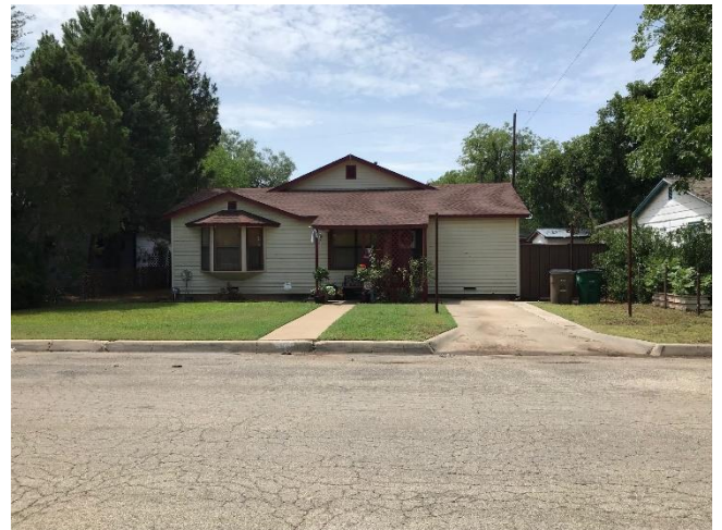
SOUTH AT SUBJECT PROPERTY (FRONT)
