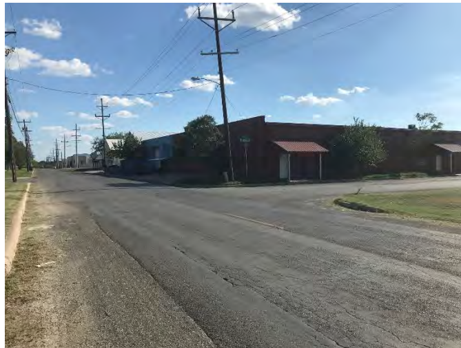
LOOKING SOUTHWEST – RUST STREET
