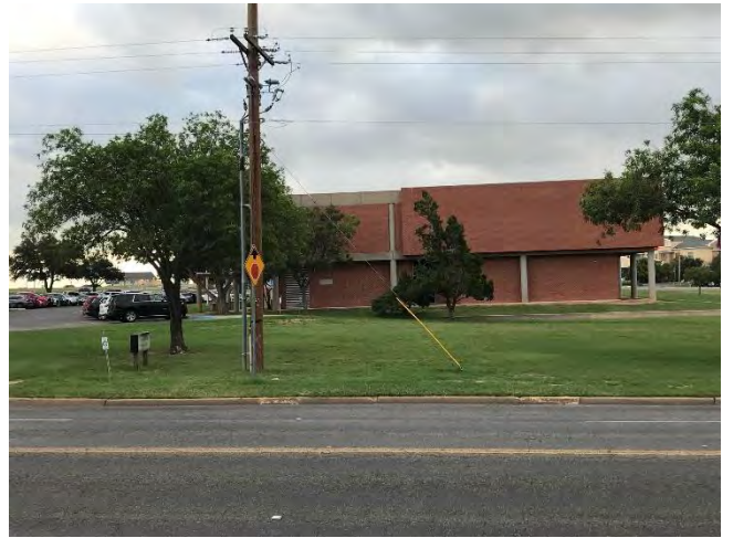
LOOKING EAST AT SAISD BUILDING (1620 UNIVERSITY)
