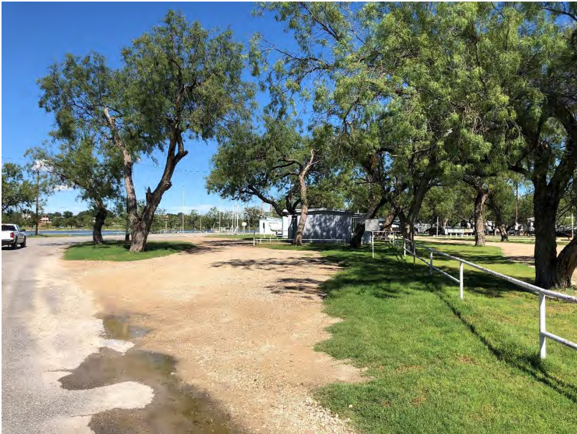
Park Restroom Facility
