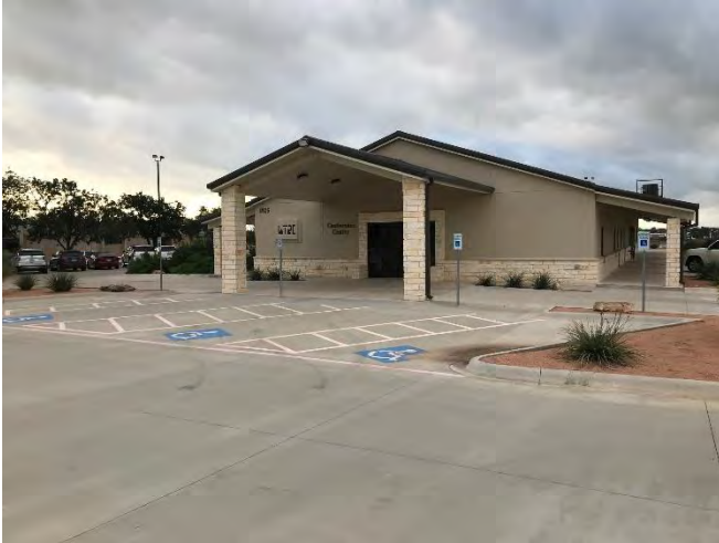
EXISTING BUILDING CLOSE-UP (1925 UNIVERSITY)
