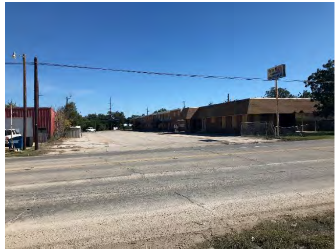
EAST LOOKING AT PROPERTY
