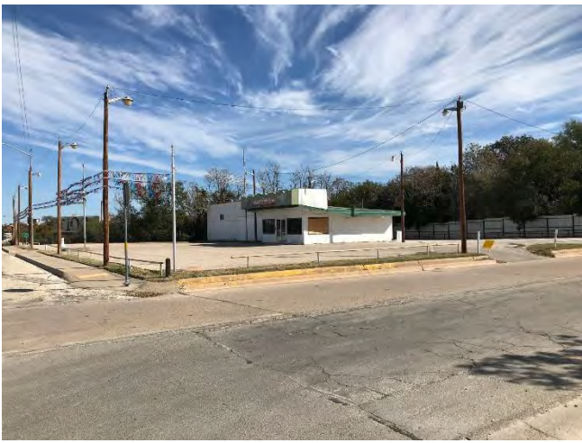
SOUTHEAST AT PROPERTY
