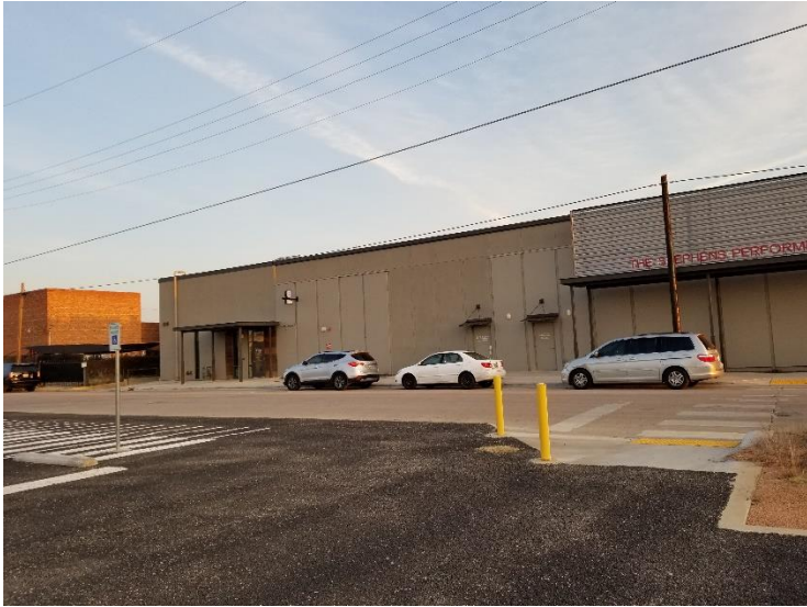
North Face of Building
