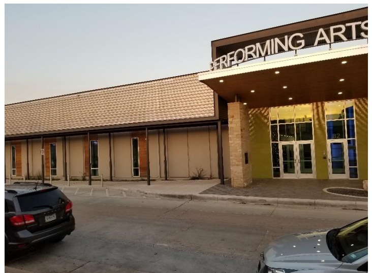
Building Front Overall
