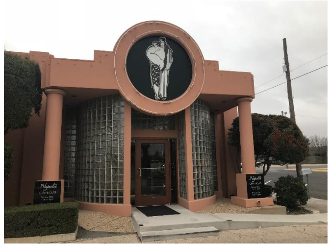
SOUTHWEST AT EXISTING BUILDING (EXISTING SIGN – NOT PART OF APPLICATION)
