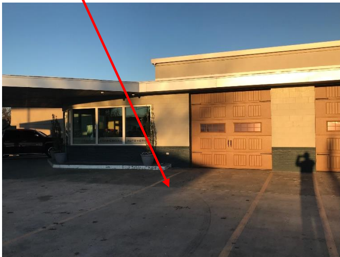
WEST AT EXISTING BUILDING (BRICK BASE)
