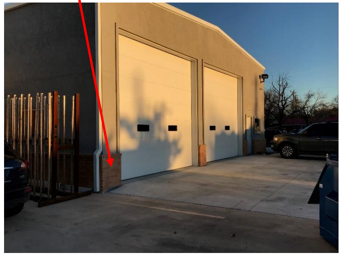
WEST AT NEW ADDITION (BRICK BASE)
