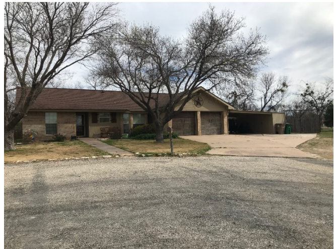
EAST AT PROPERTY
