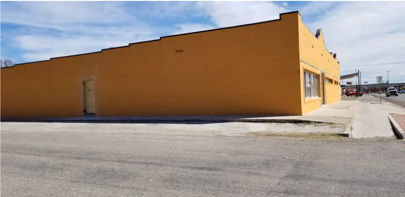
Building at the corner of 10 th Ave. and N. Chadbourne St.
