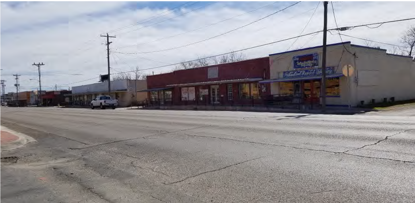
Commercial buildings across N. Chadbourne across the street from the Tortilla Factory
