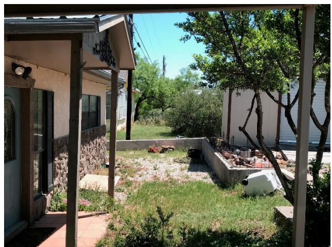
EXISTING PORCH AND ONE-STORY ADDITION
