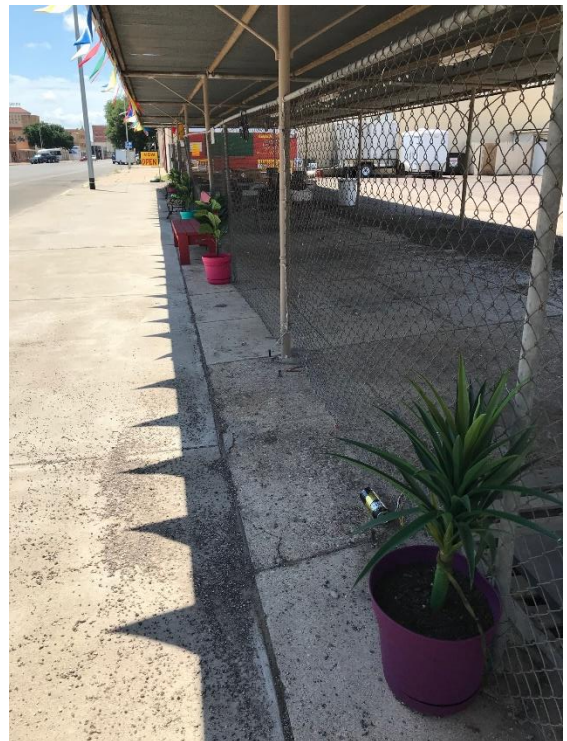
VIEW SOUTH ON CHADBOURNE STREET
