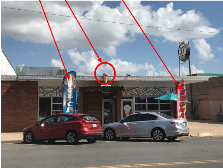
FRONT OF BUILDING (FLAG SIGNS IN RIGHT-OF-WAY AND ICE CREAM CONE TO BE REMOVED)
