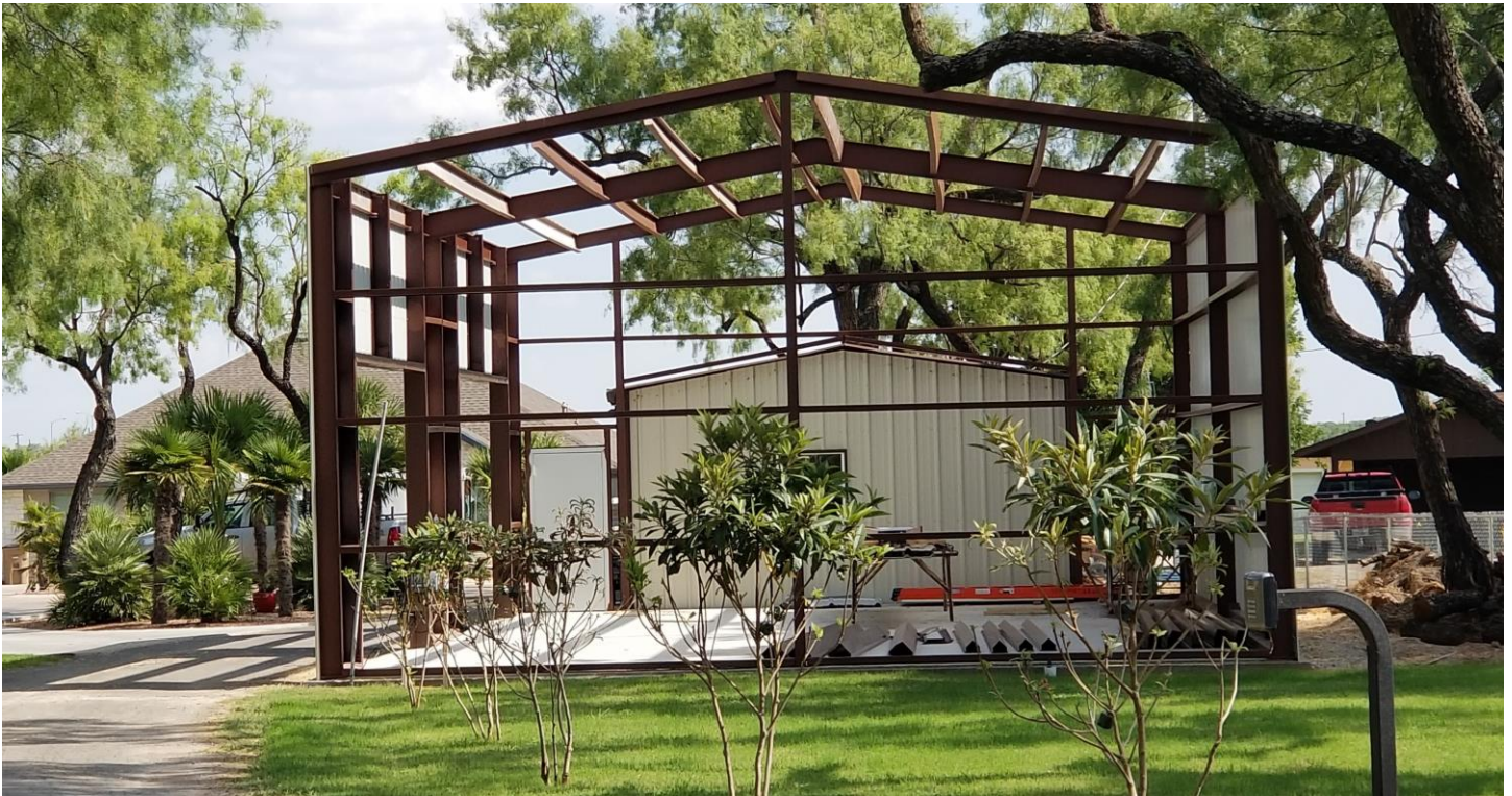
Close up of structure and placement.
