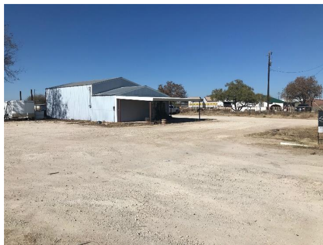
NORTHWEST AT SUBJECT PROPERTY (6993)
